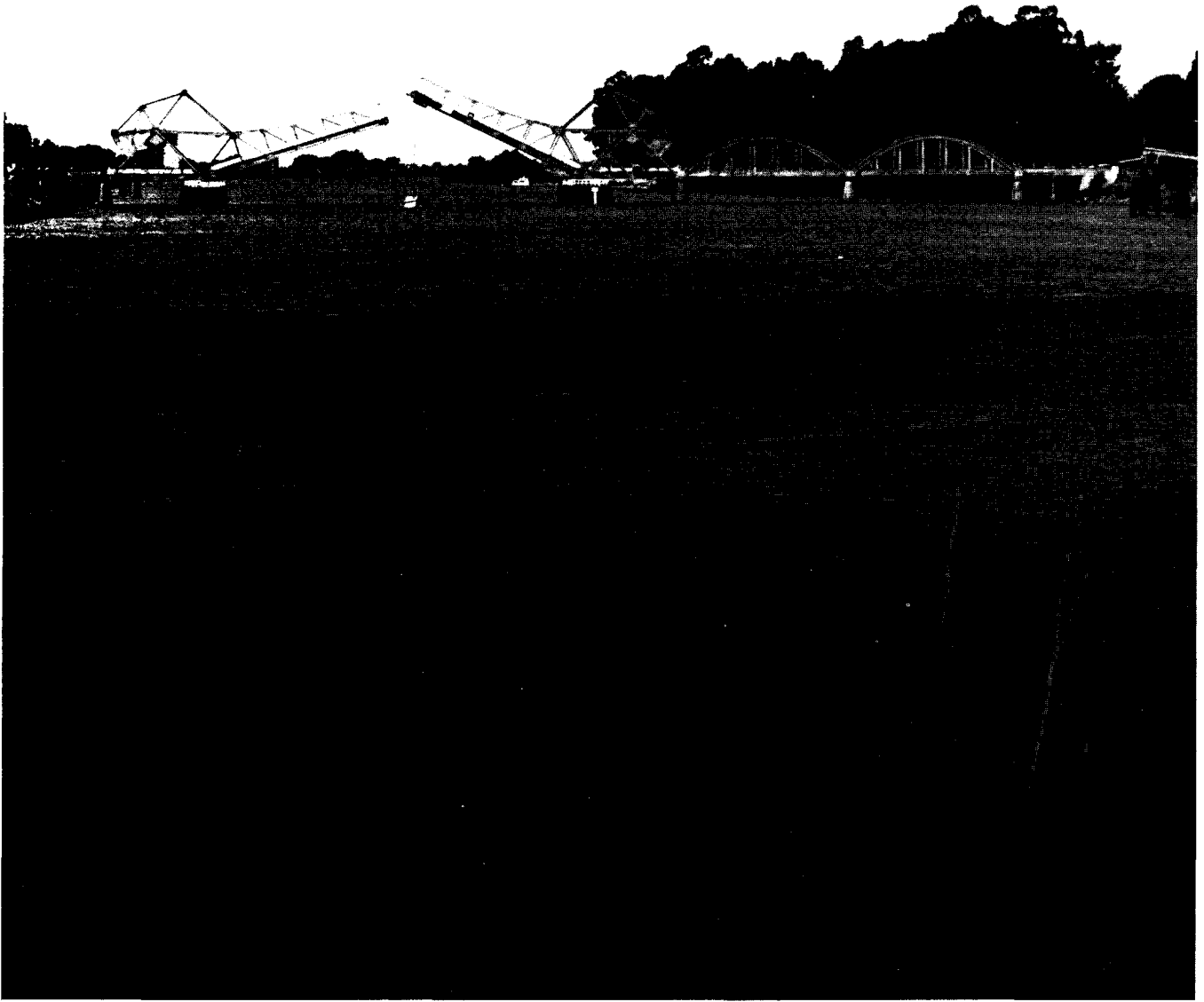
Drawbridges accommodate the mix of land and water traffic in the Delta. This bridge on Highway 160 crosses the Sacramento River near Isleton and must open frequently during the summer boating season.
