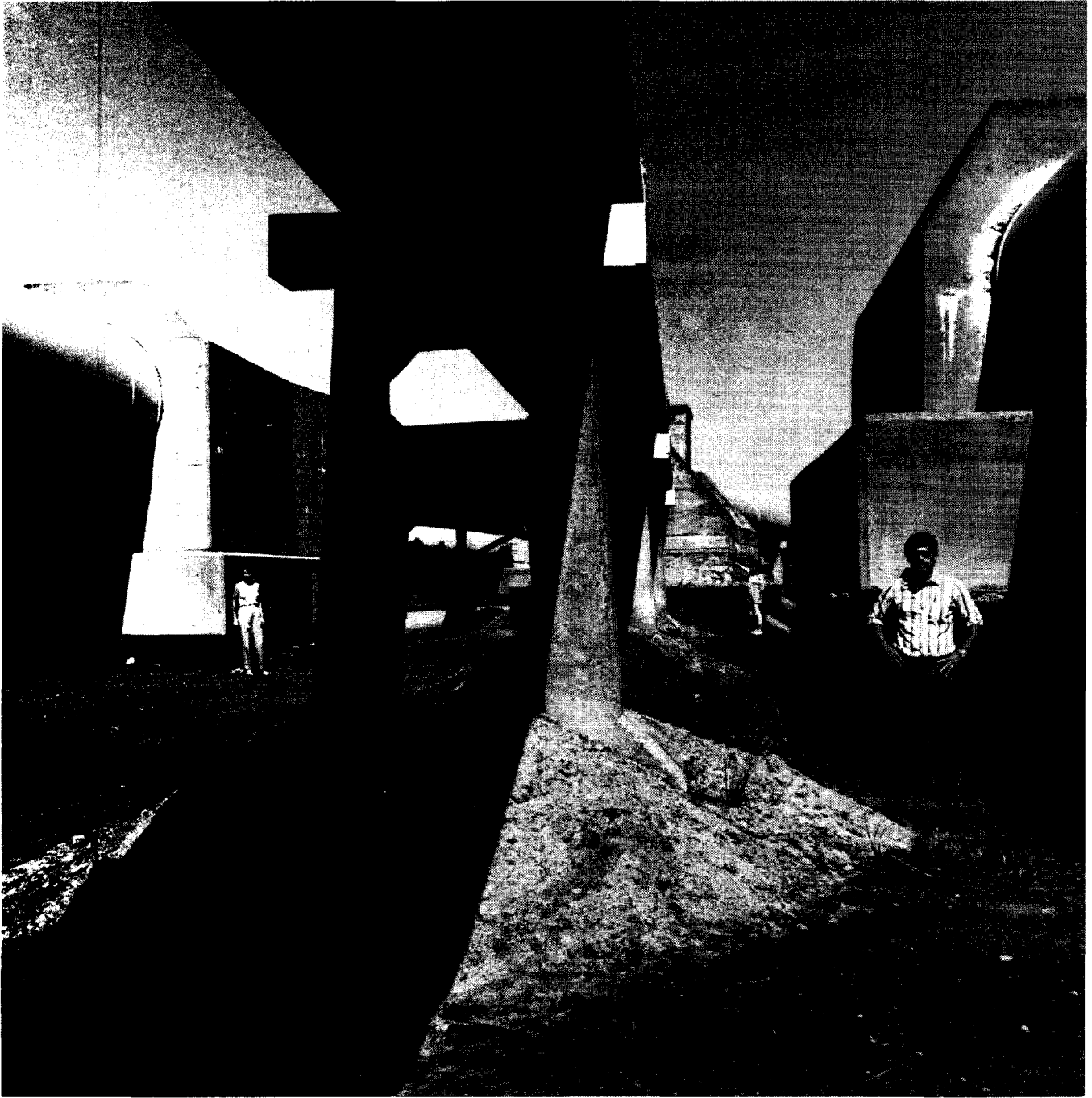
The East Bay Municipal Utility District Mokelumne Aqueduct, which crosses the Delta's peat soil, shows the amount of land subsidence since construction. These concrete anchor blocks, once at ground level, are supported by piles that extend to a firm foundation.
