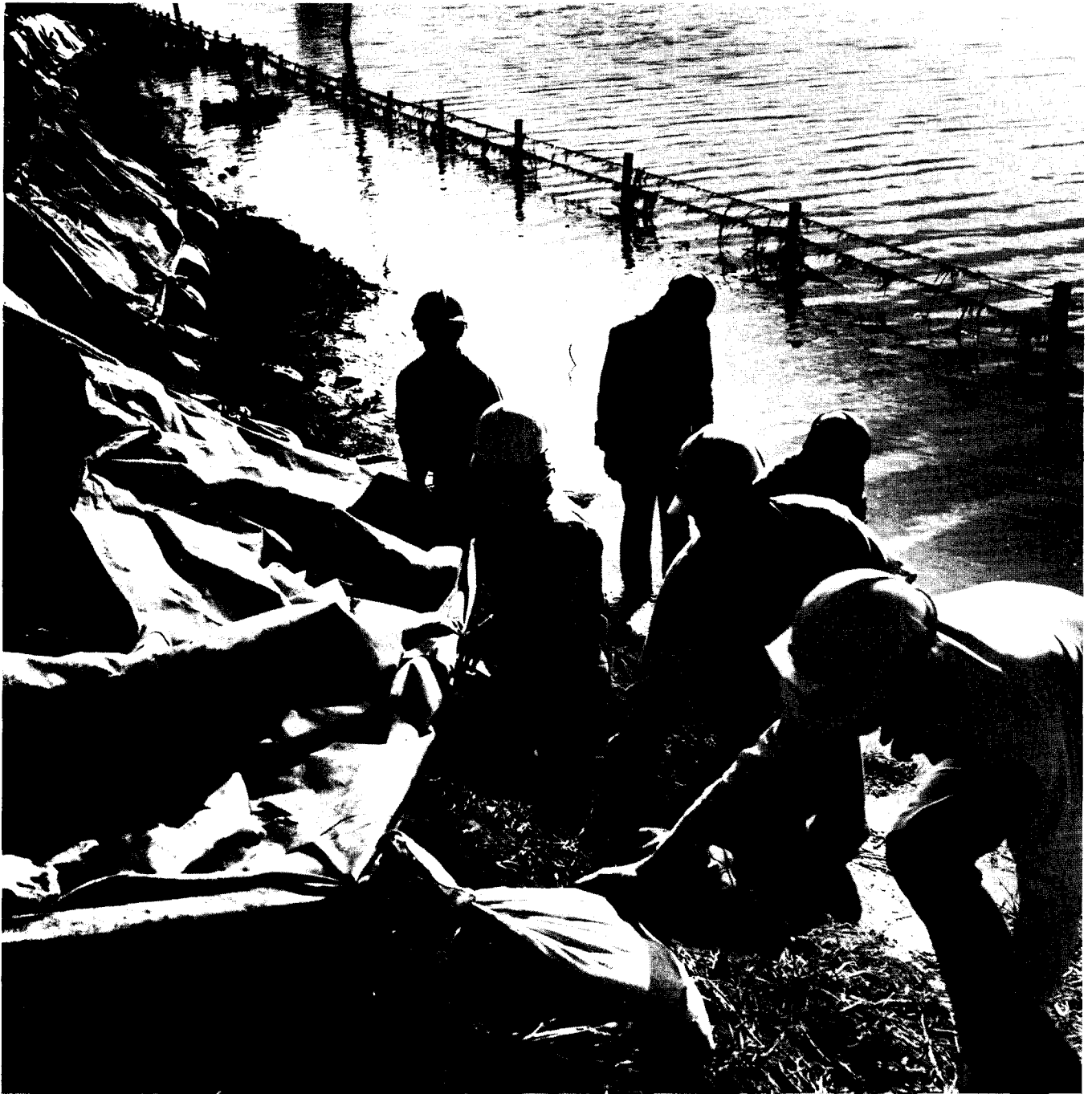
California Conservation Corps crews placed protective canvas on the landward side of this levee on Holland Tract when it flooded in 1980. Without such protection, floodwaters would soon erode the remaining levee.
