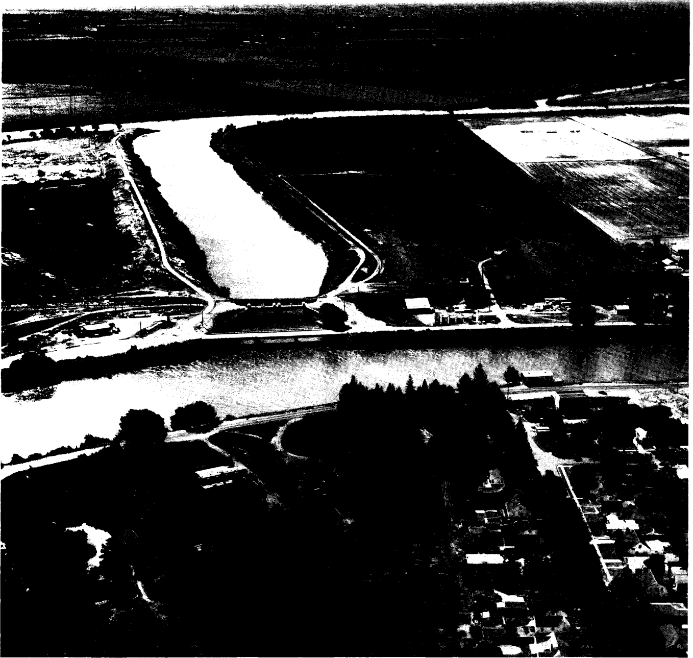
The Delta Cross Channel, constructed by the Bureau of Reclamation in the 1950s, connects the Sacramento River (foreground) with the Snodgrass Slough and Mokelumne River system (background). Water released from upstream storage reservoirs flows through the Cross Channel to interior Delta channels and the export facilities near Tracy.
