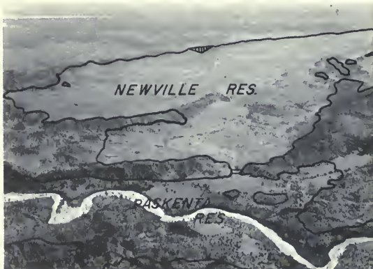
Paskenta-Newville Project, Thomes Creek in foreground
