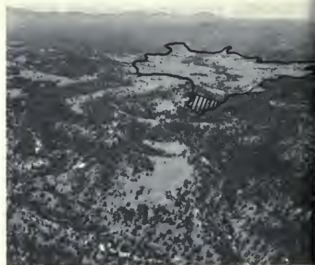
Millville Dam and Reservoir, Old Cow Creek left foreground
