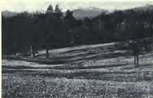
Hulen Reservoir area
