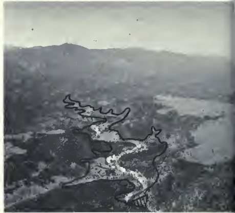
Dippingvat Dam and Reservoir
